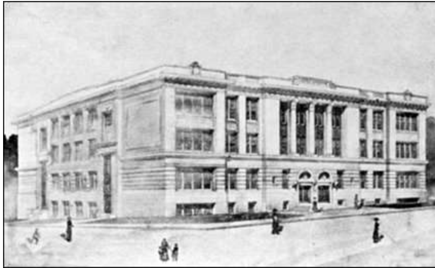
NEW QUARTER MILLION DOLLAR HIGH SCHOOL BUILDING UNDER CONSTRUCTION
