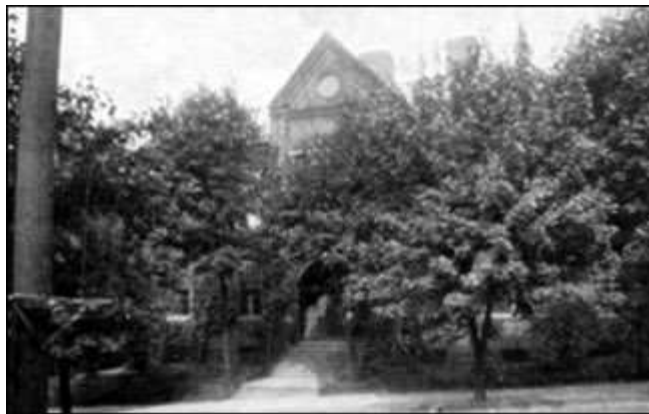
WEBSTER SCHOOL BUILDING
