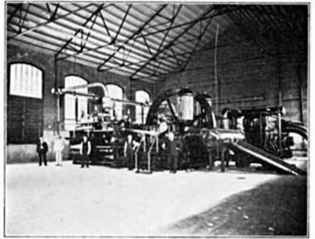
INTERIOR OF PUMPING STATION.
