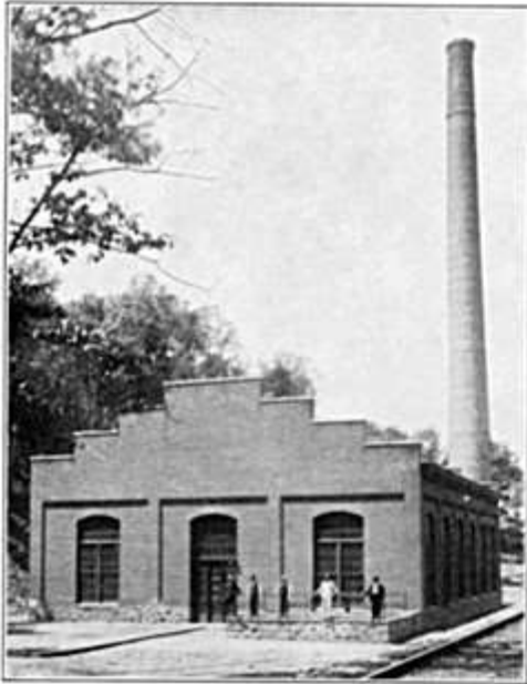
EXTERIOR OF PUMPING STATION.
