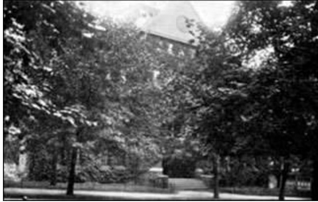
CENTRAL HIGH SCHOOL BUILDING
